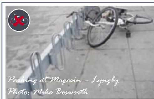
Bad rack which does not "grip" the front wheel sufficiently well. The stand is model 51 GE from Vekso.
