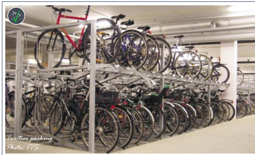
*Acceptable stand for two-tier bicycle parking solution from TTS. Access to the top tier is facilitated by a ramp which guides the bicycle into place and minimises lifting; at the same time the bottom tier is slightly sunken.*
